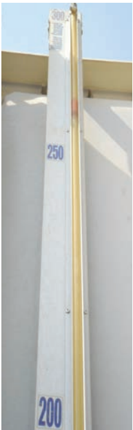
Glass clear tube level indicator
