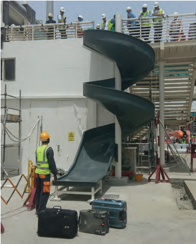
Airports Baggage Handling
