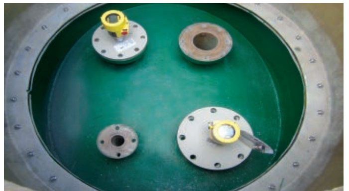
Pressure and Temp Gauge
