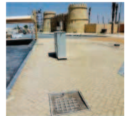
GRP recessed Manhole cover at parking area at YAS Water Park
