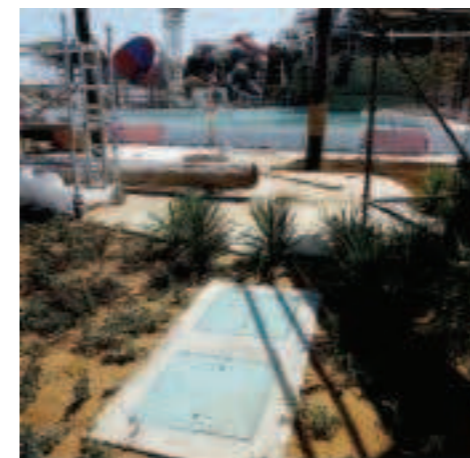
GRP Manhole covers Class A15 at YAS water park
