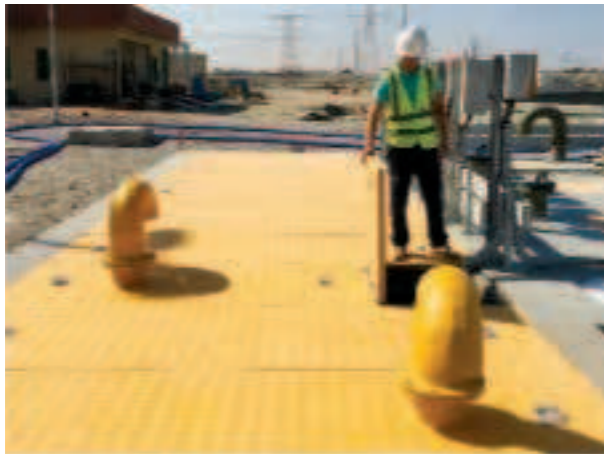
GRP flat chequered covers , design 5 KN/m2
