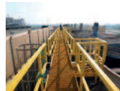
District Cooling Plant - Dubai, UAE
