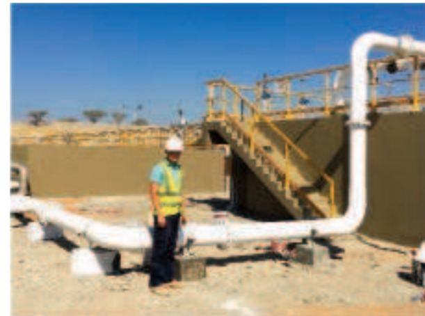
GRP safety handrail
