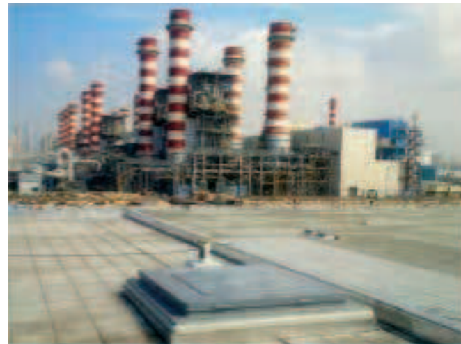
GRP roof sealed cover for Potable Water tank
