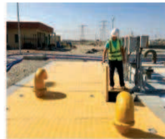
GRP Pultruded wave pool grating at Dubai Park
