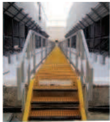
GRP Walkway at Emicool DCP at motor city
