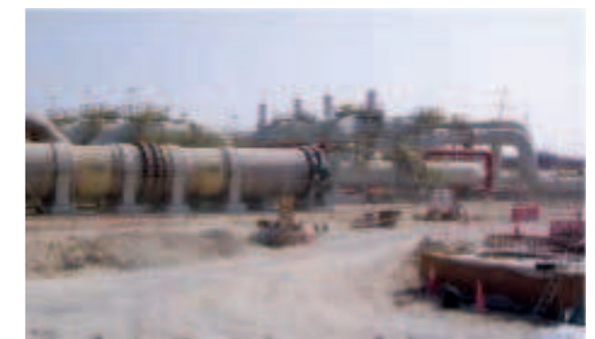
Ras Laffan Common Cooling Water System
