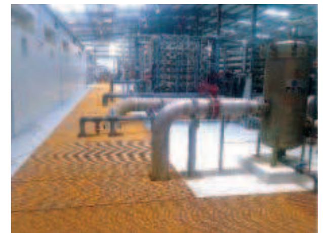
GRP Pultruded Heavy duty grating over pipe trench, 3 tons Forklift
