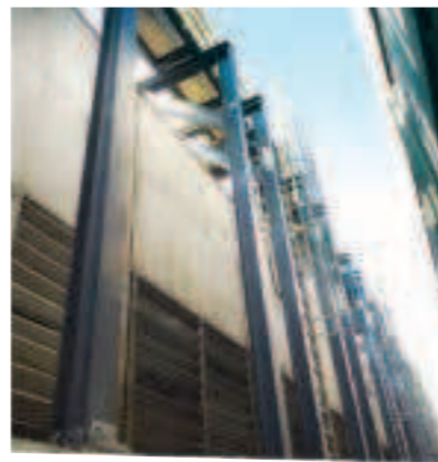
GRP column for High rise platform at Emicool DCP at DIP
