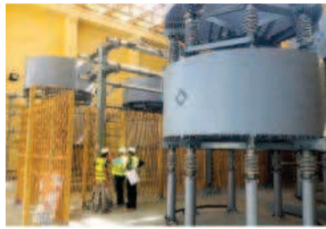
GRP grating fencing 3m High at Aweer Substation
