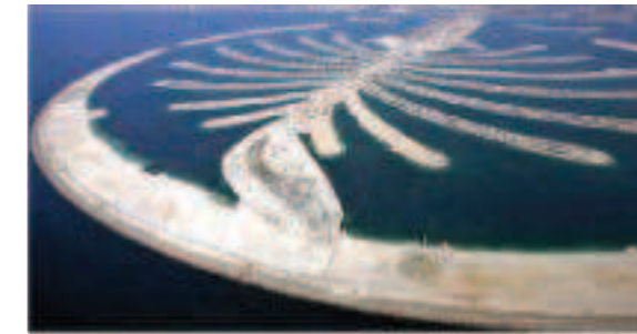
Palm Jumeirah Service Tunnel
