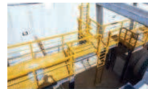
GRP U/G service platform for Valve chambers at Emirates Road
