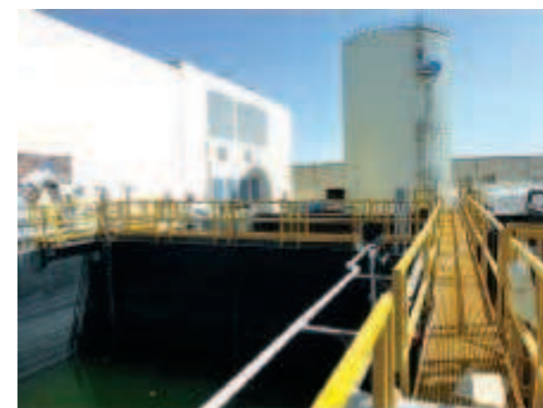
GRP walkway WWTP Riyadh
