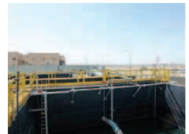
GRP Walkway WWTP Riyadh
