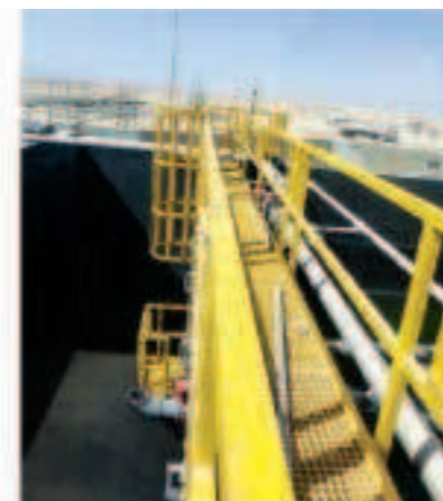
GRP walkway on Concrete wall of WWTP in Riyadh
