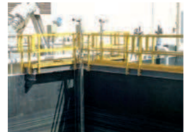
GRP walkway WWTP Riyadh
