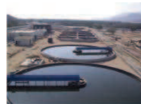
Fujairah Sewage Treatment Plant
