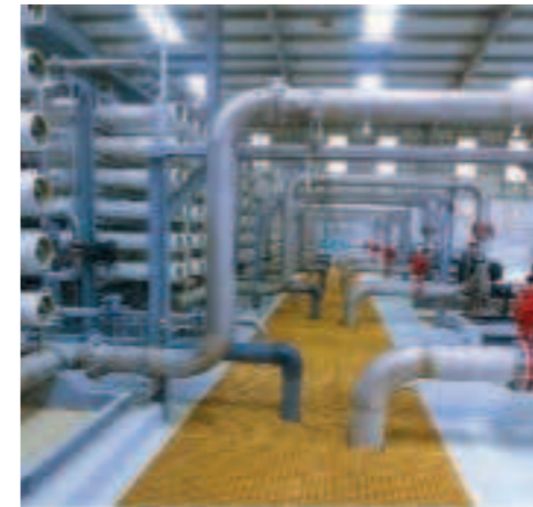
GRP molded grating SM 50x50 over pipes trench Design 5 KN/m2
