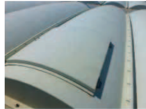
GRP self supporting curved covers , design 2.5 KN/m2
