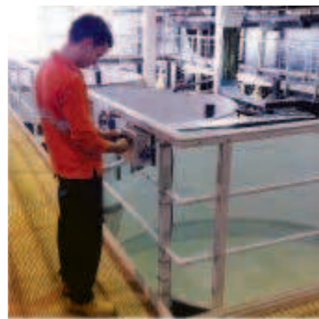
GRP handrail w/2 middle rail & kickplate
